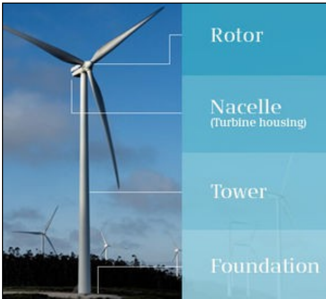
Fig 6 Wind turbine parts
