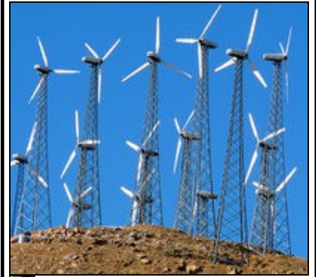
Fig 8(b) Lattice tower
