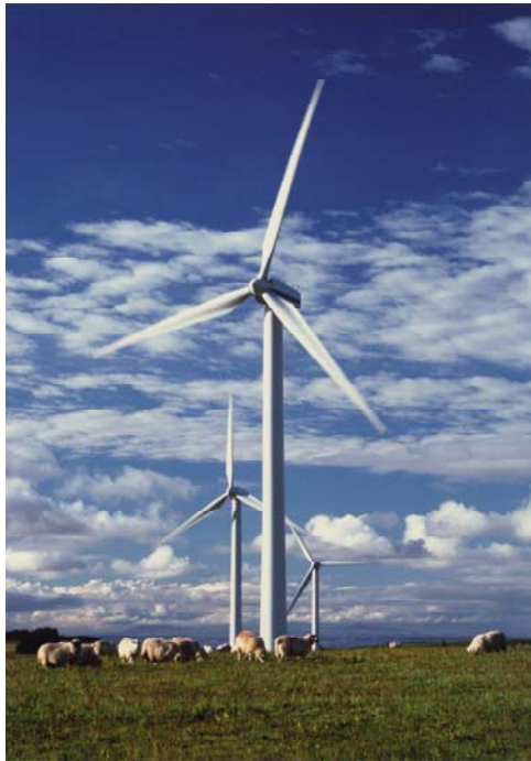
Fig. 2.3. Three bladed horizontal axis wind turbines (Hamish Hill/Courtesy of Renewable Energy Systems Ltd., www.res-ltd.com )
