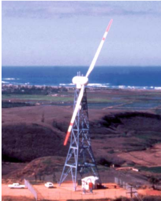
1.3. The MOD OA wind turbine (Courtesy of Hawaiian Electric Company, Inc., http://heco.com )
