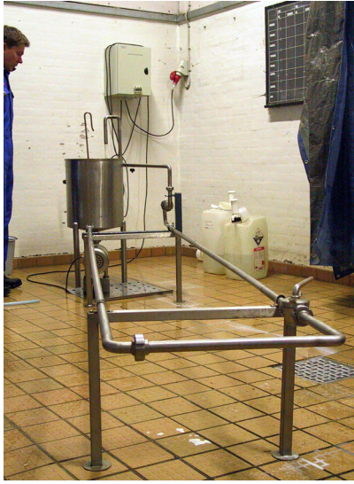
Figure 3. Picture of the pumping system used in paper II and III.
